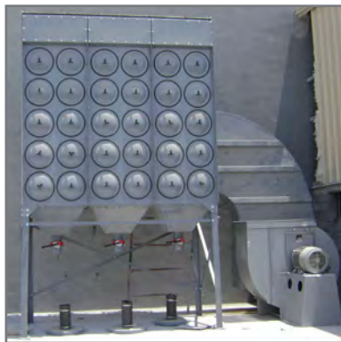
Outdoor unit, ground-mounted fan
