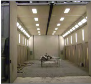
Drive-through, crane slot, manual metal doors
