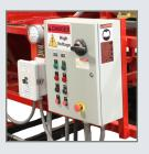
Easy-to-access control box with Emergency Stop Button for fast system shutdown.
